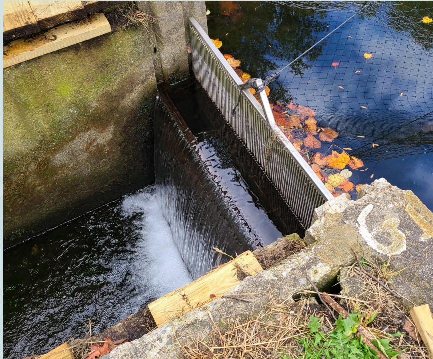
Waterfall before installing the wheel
