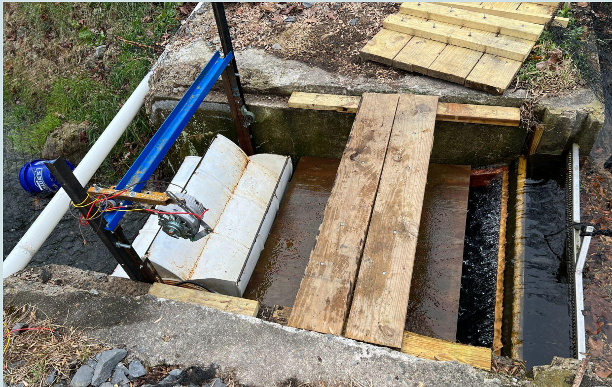
Wheel installed with alternator
