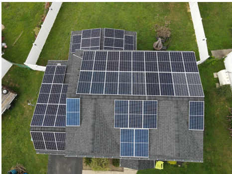
Pinnacle Exteriors Solar Installation; Levittown, PA
