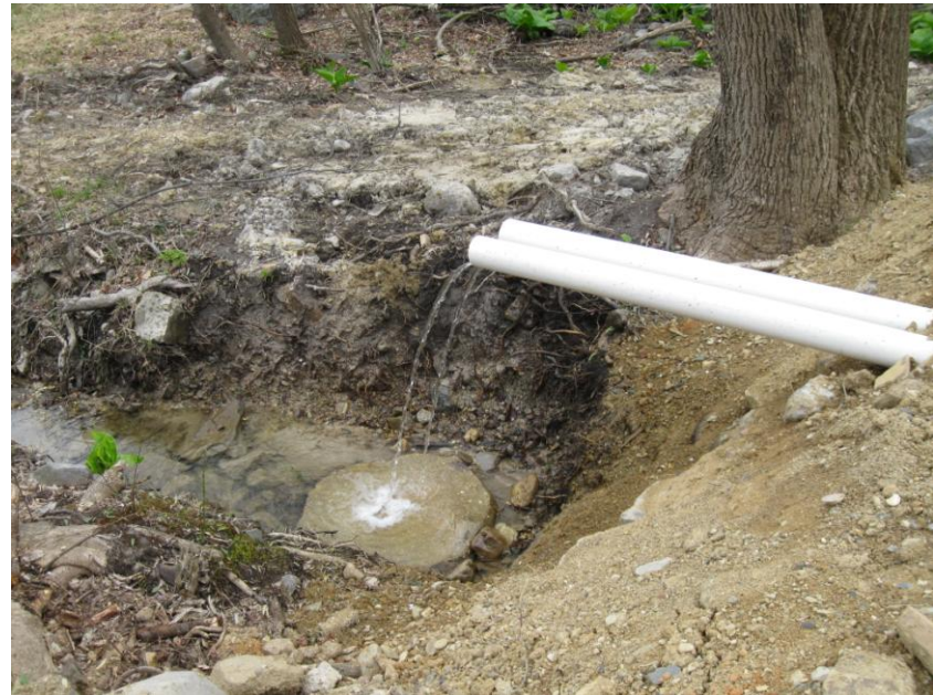
Waterfall constructed based on the recommendation of the Tech Clinic
