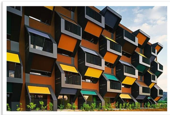
Housing complex in Slovenia that is a series of honeycomb modular apartments Source: inhabitat.com
