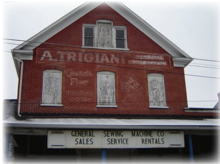
Fig. 64: Historic building in need of restoration in the Slate Belt.
